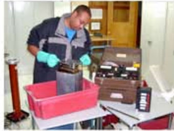
Repair of Hipot transformer tank - Calibration and certification.
