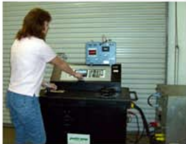
Multi-amp circuit breaker test set max 100,000 amps - Preventative maintenance, calibration and certification.
